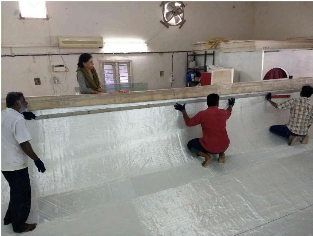
Figure 8: Quadraxial fibre layer in position in preparation for the vacuum infusion.
